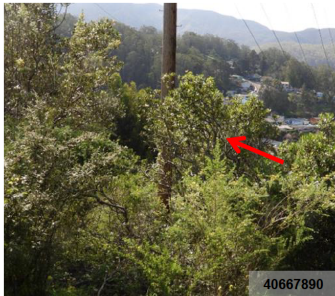
Trees and woody brush at base of pole, blocking pole access/climbing
