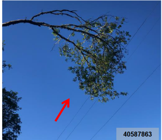
Tree contacting conductors
